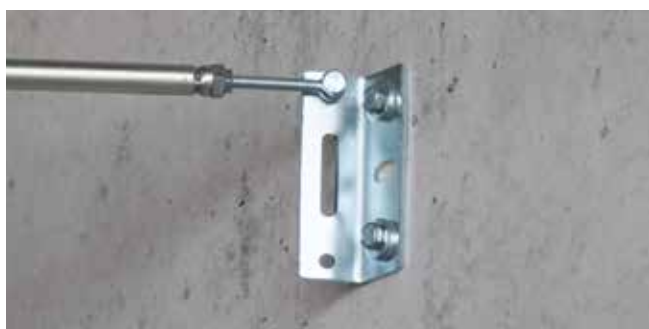
Fixing of brackets and console bearers
